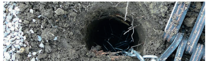
Small hole in ground for anchor chains + point foundation (ca. Ø 5.00 cm)
