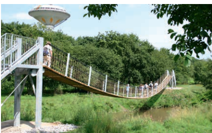
Wooden walkway bridge, Length 54 m
