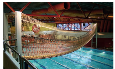
Net tunnel in V-Form (Swimming pool area), Length 21 m
