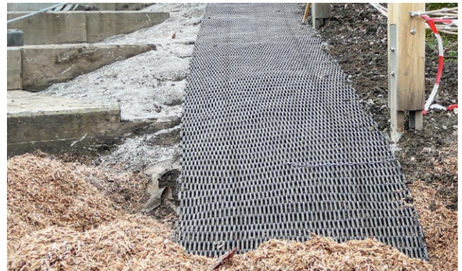
Mat directly after placing
