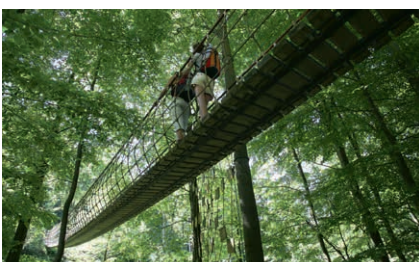
Wooden walkway bridge, Length 40 m
